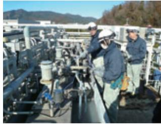
Trainings are held by setting accidents assumed for each facility and equipment owned. Procedures to stop or replace in case of malfunction of a valve of the wastewater treatment facilities are confirmed.
